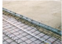
Start pouring / placing the concrete
