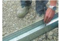
Insert fixing pegs at 600mm centres
