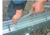
Install PVC capping strips onto units
