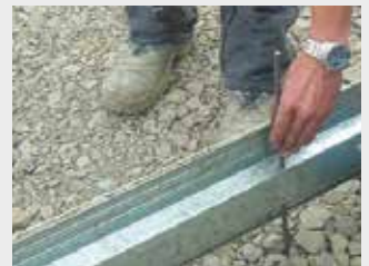
Insert fixing pegs at 600mm centres
