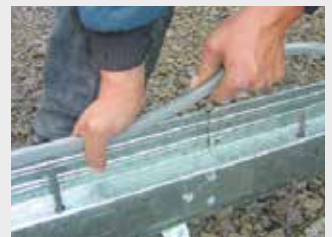
Install PVC capping strips onto units
