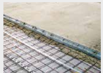
Start pouring / placing the concrete
