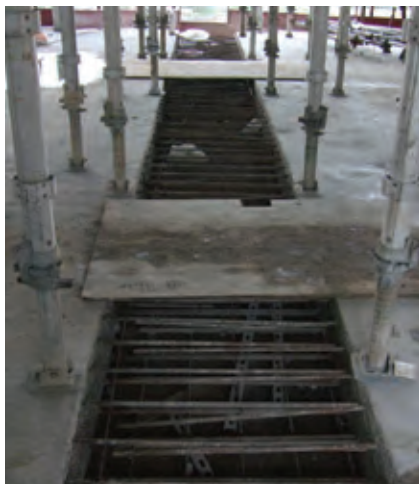
Pour Strips restrict site access, cause a trip hazard and delay progress on site
