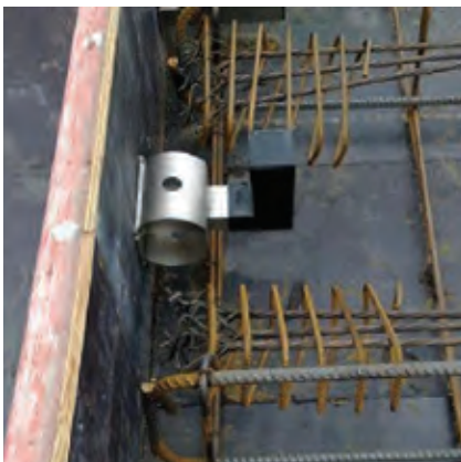
HLDQ-L30 Sleeve nailed to formwork
