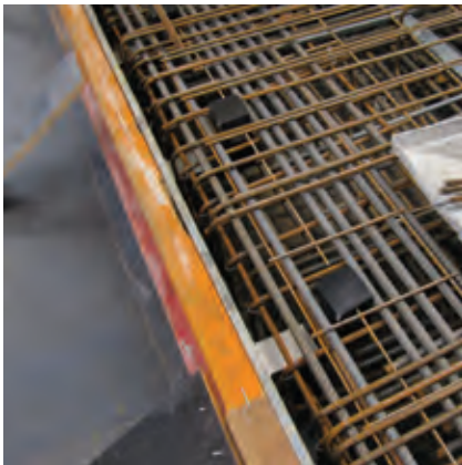
Reinforcement being located around ESDQ-L20 Sleeves
