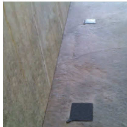
Void formers shown at Slab-to-Wall joint
