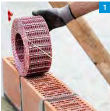
1 Apply Murfor® Compact I to the blocks.
