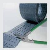
Unroll shuttering strip and cut to length with snips or angle grinder.
