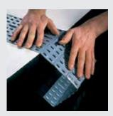
Fold shuttering strip over the edge of a table at the required length and trim.
