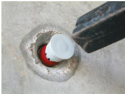
2. Hammer the Solco Form-Tie Plug with light blows from a hammer until flush with the end of the conduit sleeve
