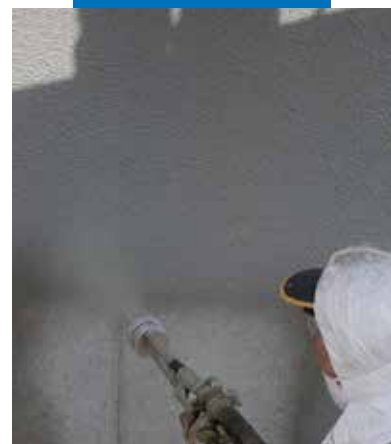
Example of Mapelast applied on a viaduct by spraying
