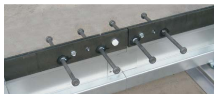
Lap joint with plastic screw
