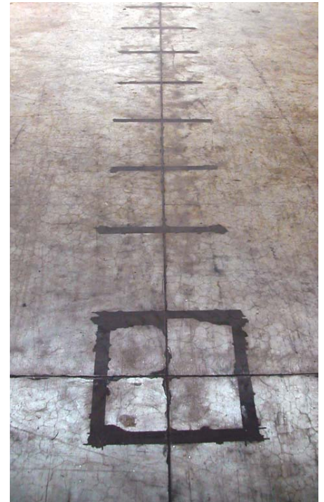
Refurbished saw cut joint with supplementary dowel bars.
