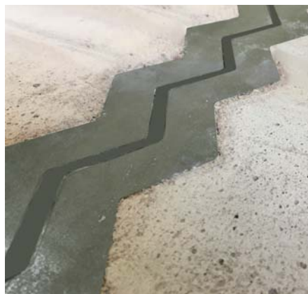
Joint expansion after shrinkage
