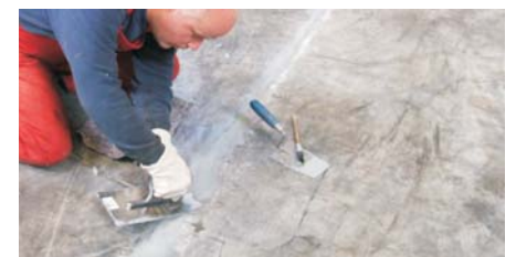
Spalling caused by the passage of handlift truck traffic once the joint opened.
