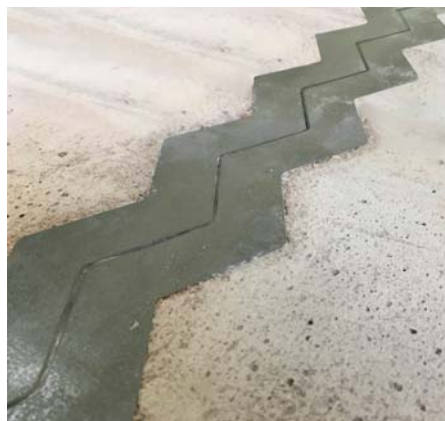
Joint after concreting
