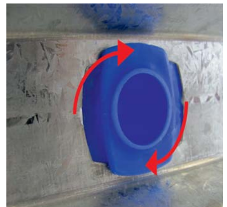
Attachment of the dowel sleeve
