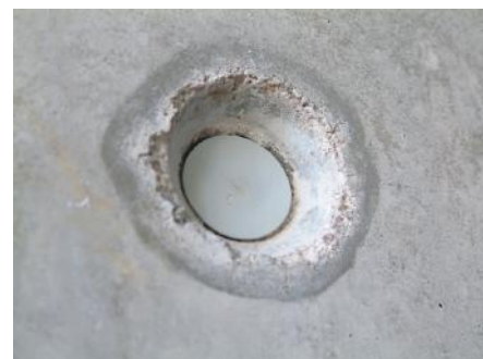
3. Solco Form-Tie Plug installed. No further finishing is required.
