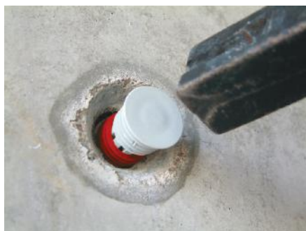
2. Hammer the Solco Form-Tie Plug with light blows from a hammer, until flush with the conduit sleeve.
