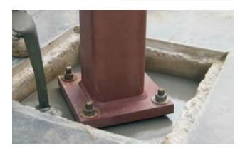
For a trowelable consistency, 25kg of the grout powder should be added carefully to 3-3.25 litres of water, progressively mixing until the required consistency is achieved. Small quantities can be mixed by hand, care being taken to accurately measure the water.
