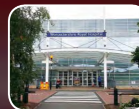
Royal Worcester Hospital, PFI Project
