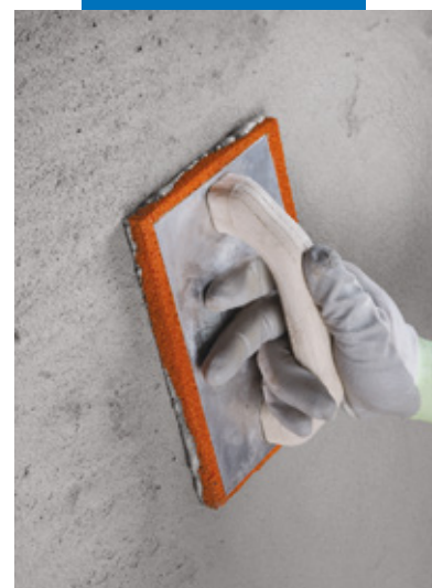
Tamping Planitop Smooth & Repair R2
