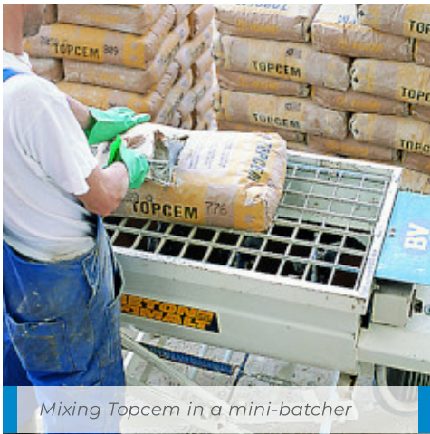
Mixing Topcem with an automatic pumping unit
