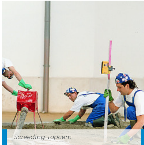
Mixing Topcem with an automatic pumping unit
