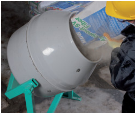
Preparation of the Mapegrout SV Fiber mix
