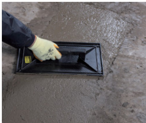
Tamping Mapegrout SV Fiber
