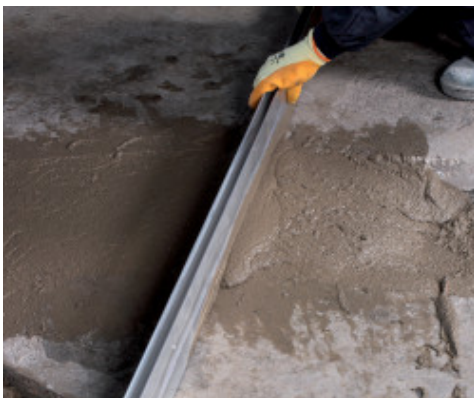
Levelling off Mapegrout SV Fiber with a straight-edge
