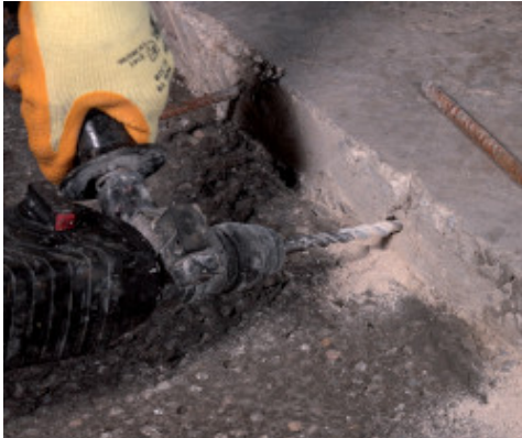
Preparation of the holes to insert the reinforcement rods (dowelling)
