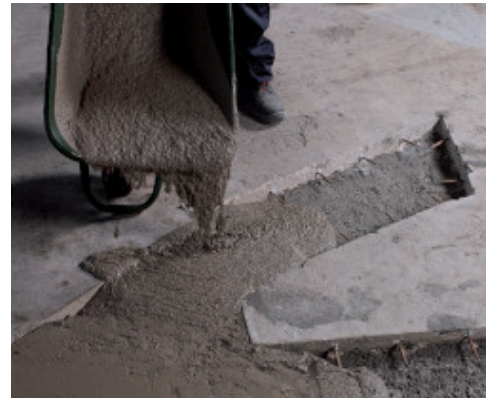
Application of Mapegrout SV Fiber in the area under repair
