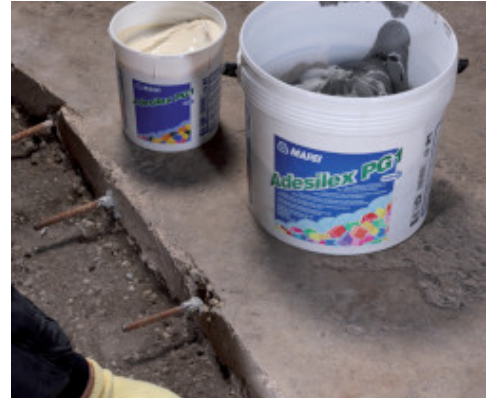
Fixing reinforcement rods for the dowelling in place using Adesilex PG1
